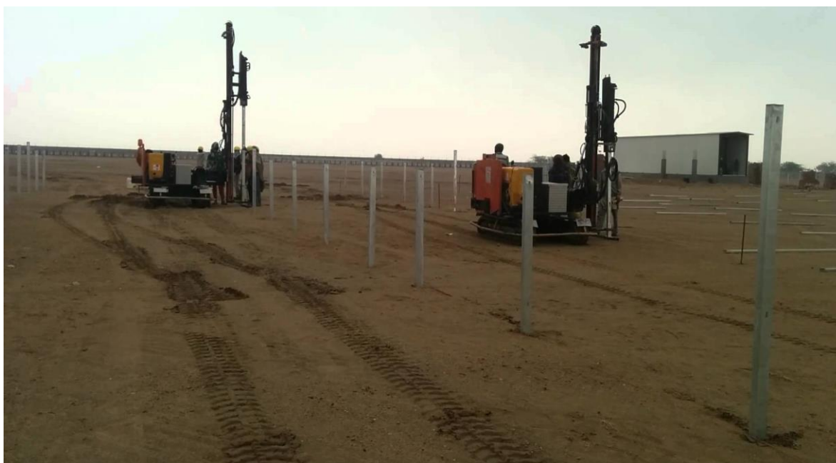
Figure 6-13: Ramming of Vertical Steel Post
